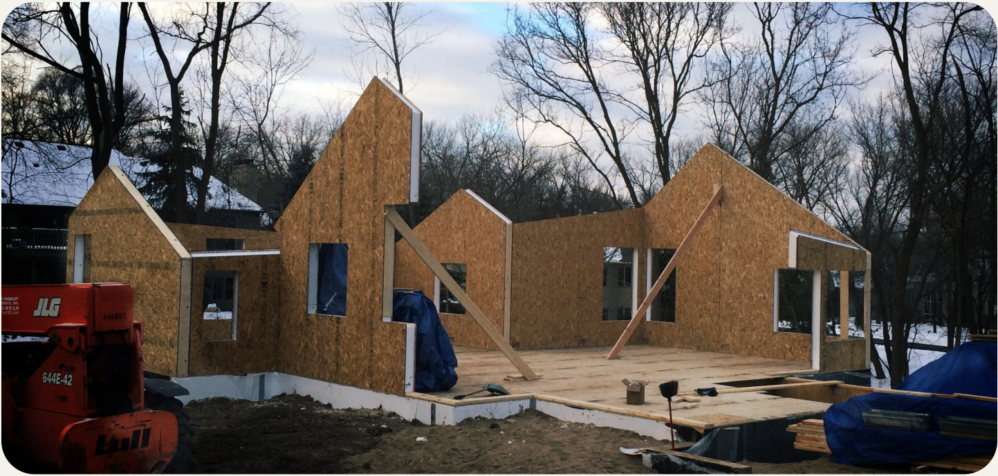
SIP Construction on the Minneapolis barnHouse
