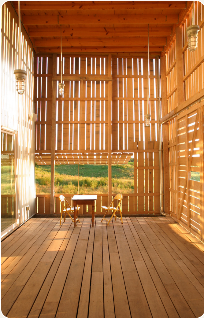
The Blair barnHouse features the barn skin pulled away from the main house to create a west-side porch and "lantern".
